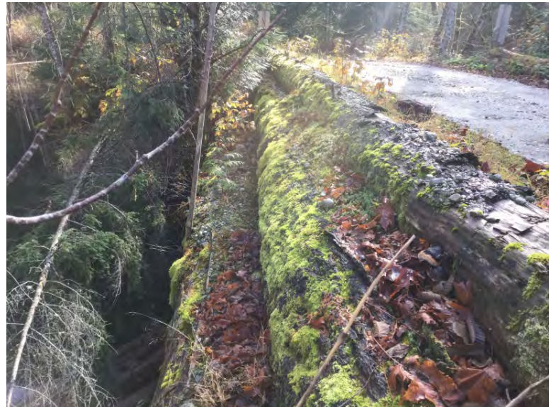
Stringers over stringers
